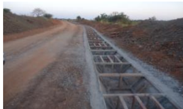
L: A section of a canal filled with water; R: A section of a canal under construction of Olweny irrigation scheme in Alebtong district
