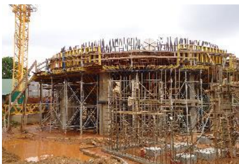
L: Anaerobic sludge digester; Kampala
