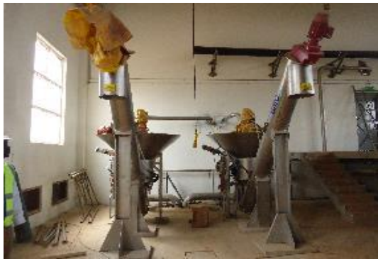
L: Grit washer; R: Sludge thickening and watering building at the NWWTP in Bugolobi, Kampala
