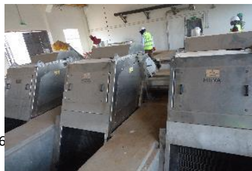
R: coarse screens at NWWTP Bugolobi
