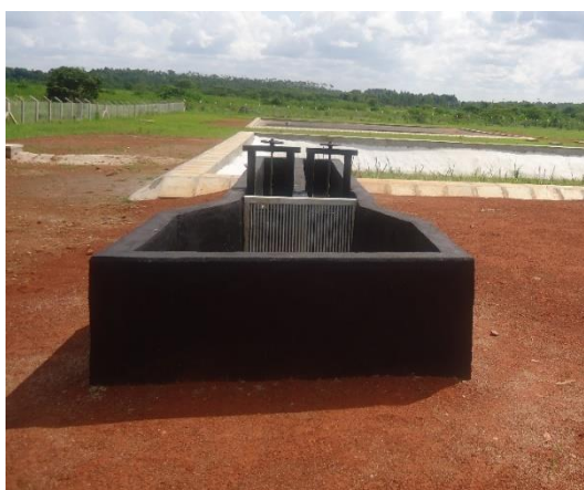
L: Fecal Sludge receiving chamber;
