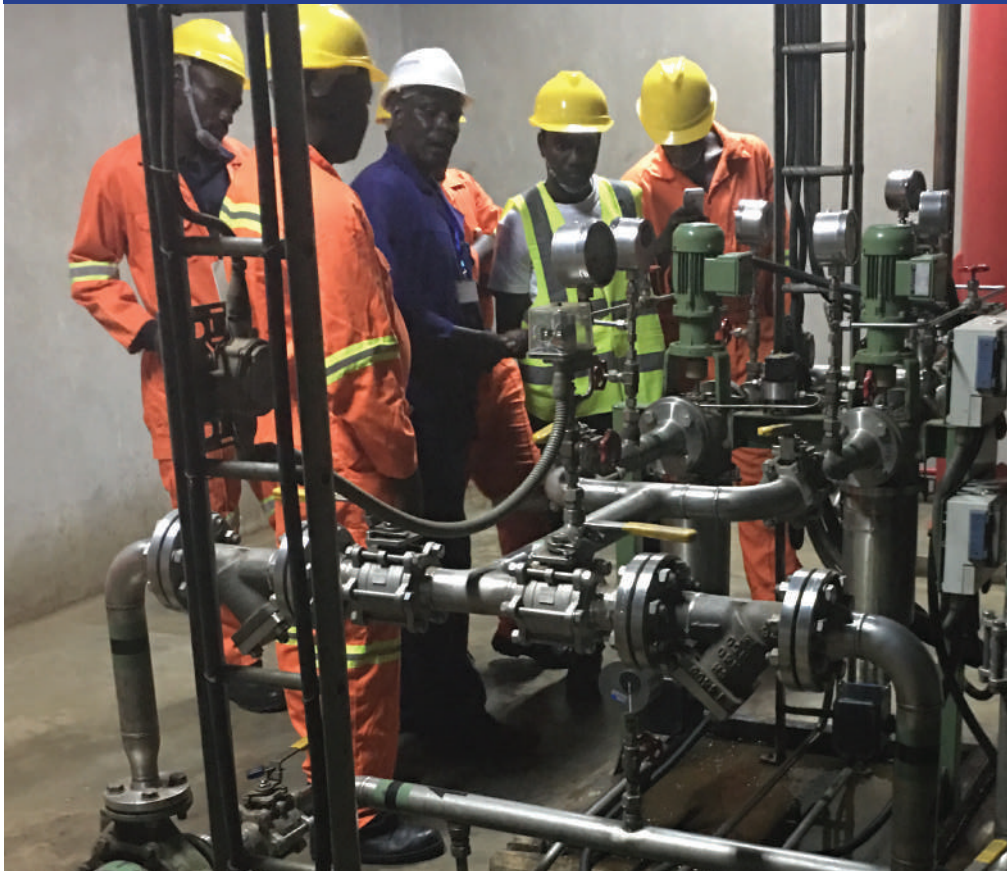
An Eskom engineer and UEGCL engineers discussing shaft seal system piping system
