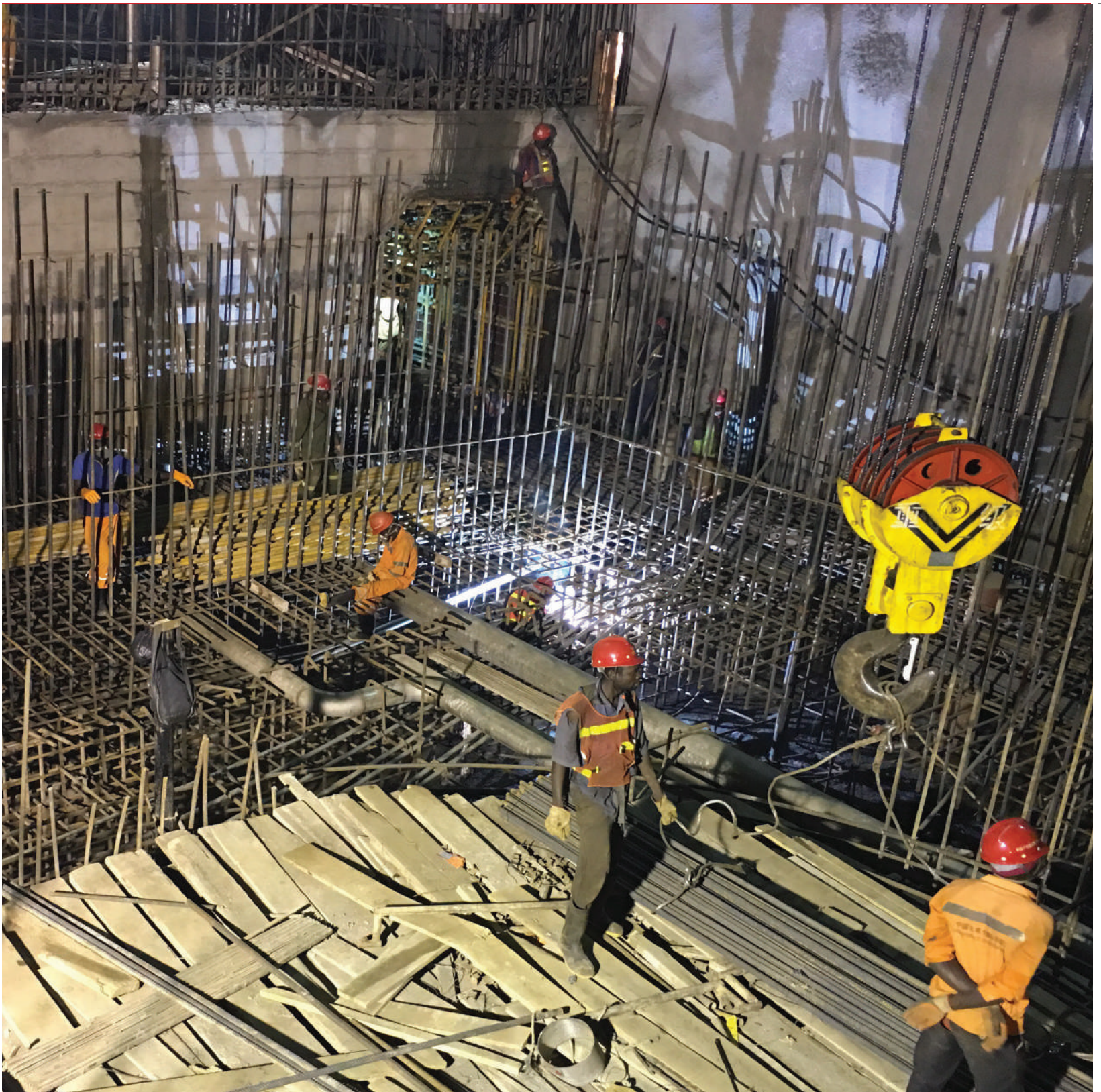
Steel form-works in the draft tube section of the Karuma hydro Power project
