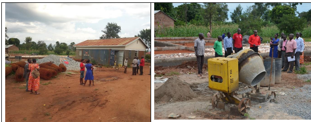
Kiyunga HC II in Kisozi Subcounty, Kamuli District was elevated to HC III following petitions from CODAID partners. It will have staff quarters, OPD and maternity, serving a population of about 20,000 people. The HC Compound had many blocks and was supply centre for other promoted HCs in the region, namely Mbulamuti 3; Nakadula 4; Buluya 2; and Kiyuga HC II.
