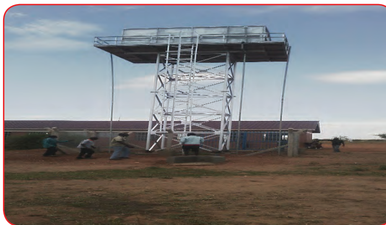
Newly commissioned clean community water project in Longariama village, Nawaikorot Parish, Ngoleriet Sub-county, Napak District
