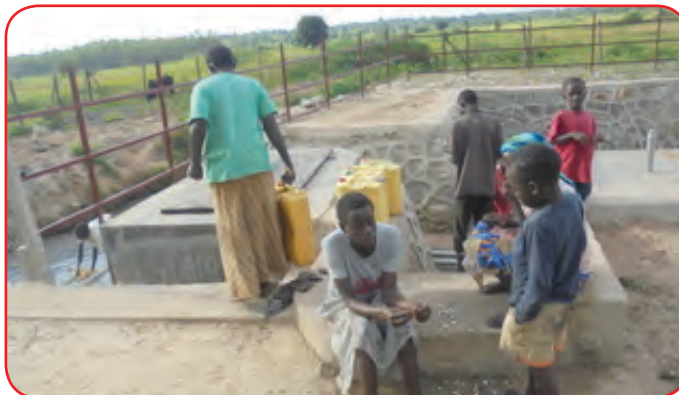
Underground water tank (Left) and newly installed Overhead water reservoir (Right) on Mukongoro Rock, May 2016
