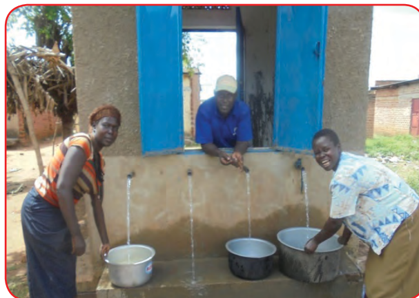
(Left) Women drawing water at Mukongoro market from a new Mukongoro Water project completed in 2016; (Right) A new water connection to Mukongoro HC III in 2016
