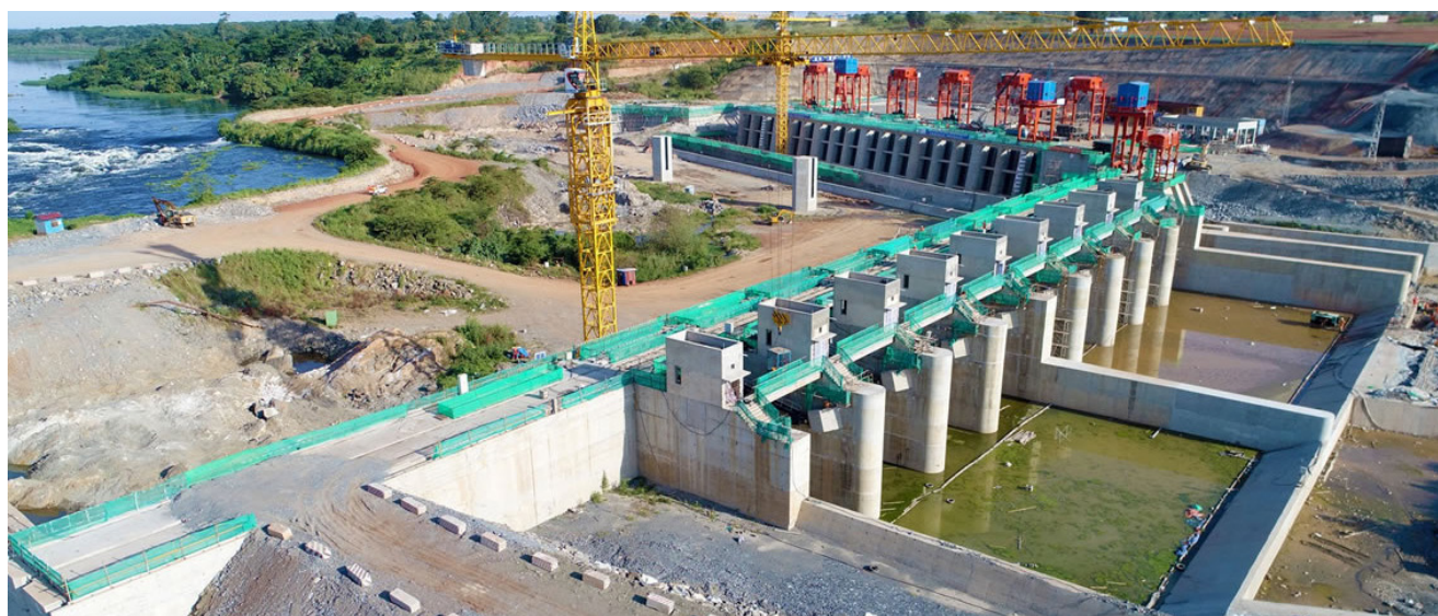
An Ariel view of the US$1.7 Billion Karuma Hydro power project under construction (85% Loan China)
