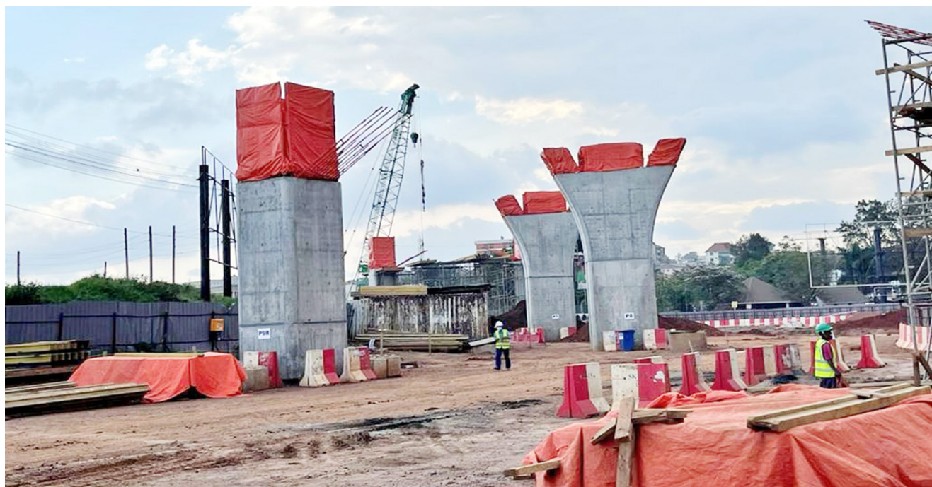
Ongoing works at the Site of construction of the sh295 billion first phase of the Kampala Fly Over project. (Photo credit UNRA)
