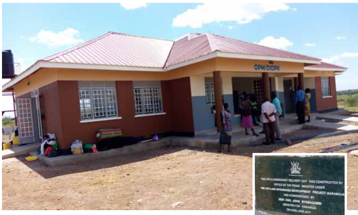
Figure 3: Health Centre 2 Constructed in Napak District by Drylands, an international NGO
