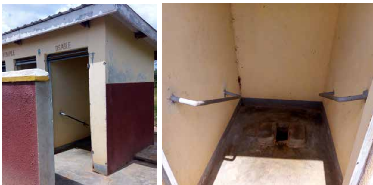
Figure 4: Latrine at Napak DLG segregated by gender and one stance adapted to cater for PWDs
