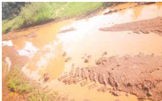
Kyema, Kiswata – Nyakitibwa feeder road before CBMs' intervention
