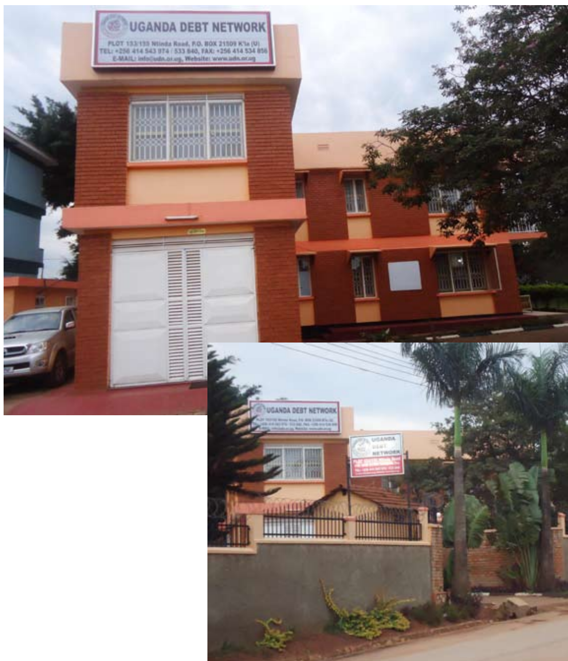
The new UDN Secretariat premises on Plot 153/155 Ntinda Road, Ntinda along Ntinda-Nakawa Road in Kampala
