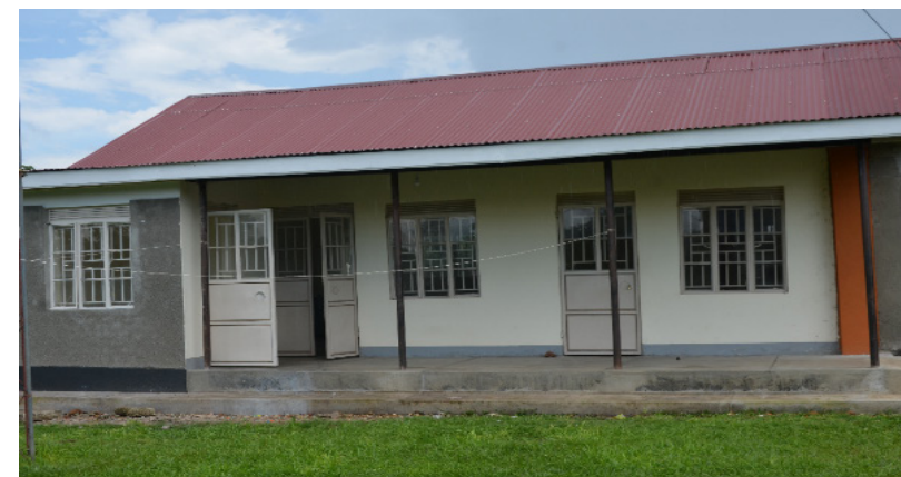
A Covid-19 isolation Centre constructed at Rugazi Health IV, Rubirizi district (Source: Pictorial from Primary data)
