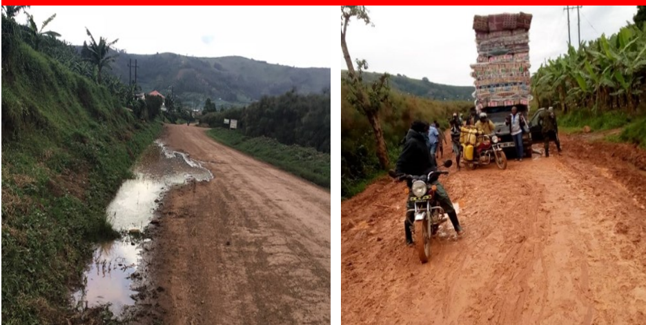
First Picture: A section of Muhanga-Kisiizi road before construction. 2nd Picture(Right) : Motorists stuck on the muddy Muhanga-Kisiizi road after it was poorly constructed with no
