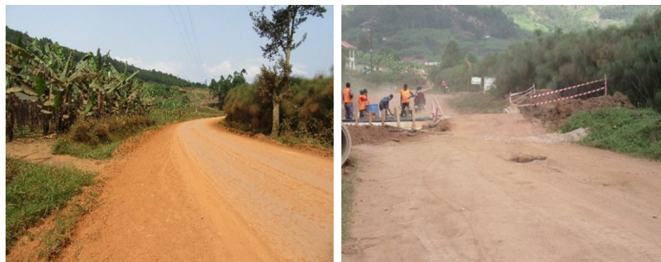
The re-constructed Muhanga-Kisiizi road and (Right Photo) workers of Greenstone Investments Ltd fixing culverts along the Muhanga-Kisiizi road .
