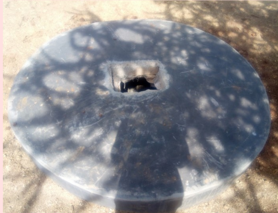
Newly constructed placenta pit of Morulinga health center ii.
