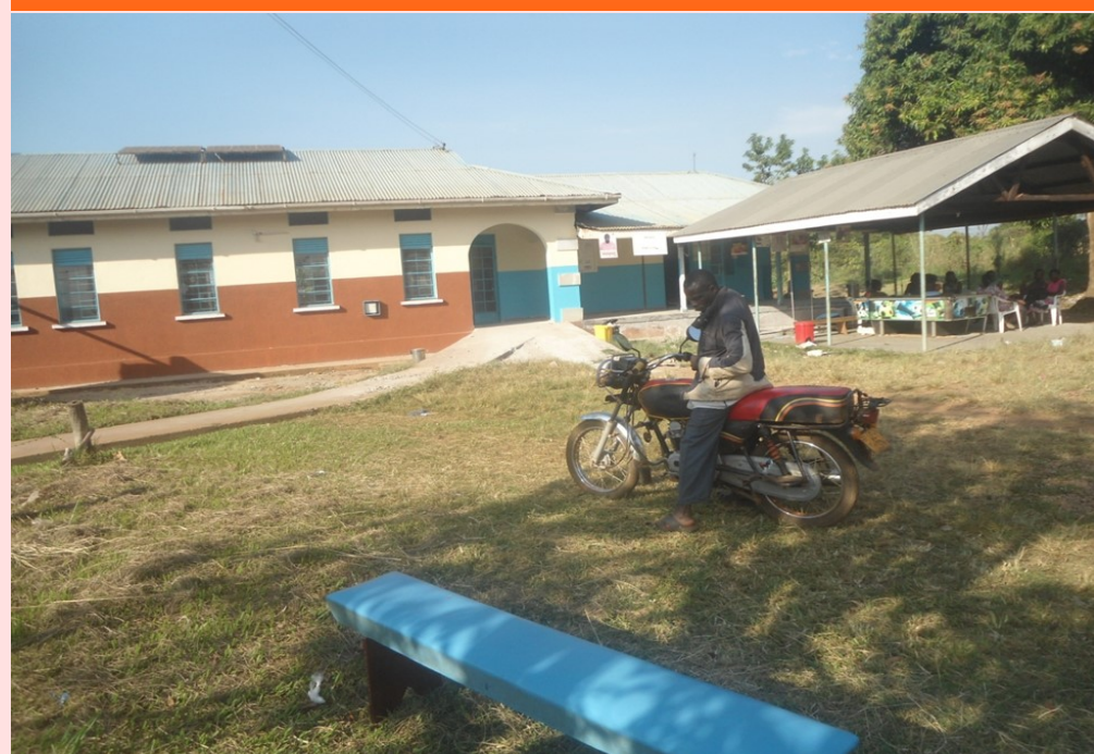
A renovated maternity ward and a theatre at Namwendwa HC IV
