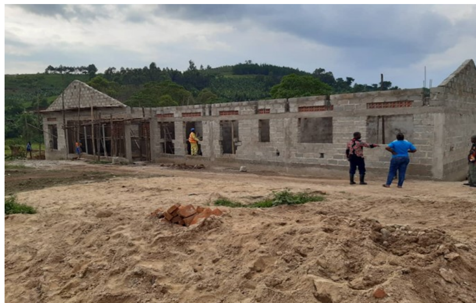
New structure at Bunyonyi health center III under construction
