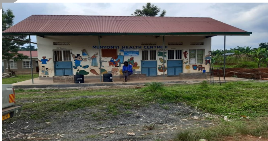
The old structure at bunyonyi health center III .
