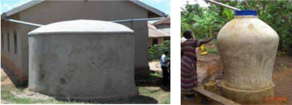
**Figure 3: Ferro-cement tank (left) and cement mortar jar**
