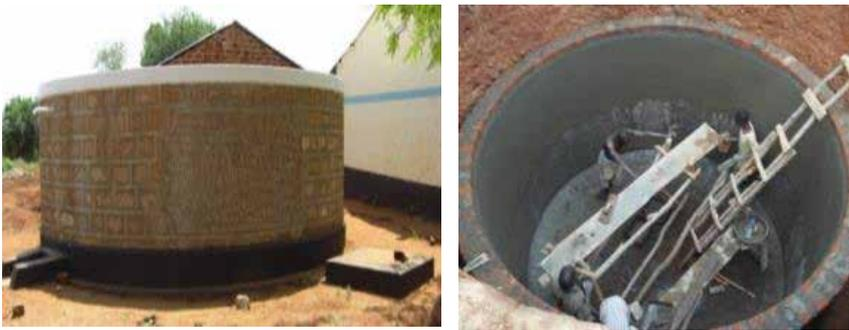
**Figure 4: Above ground masonry tank (left) and below ground tank under construction**
