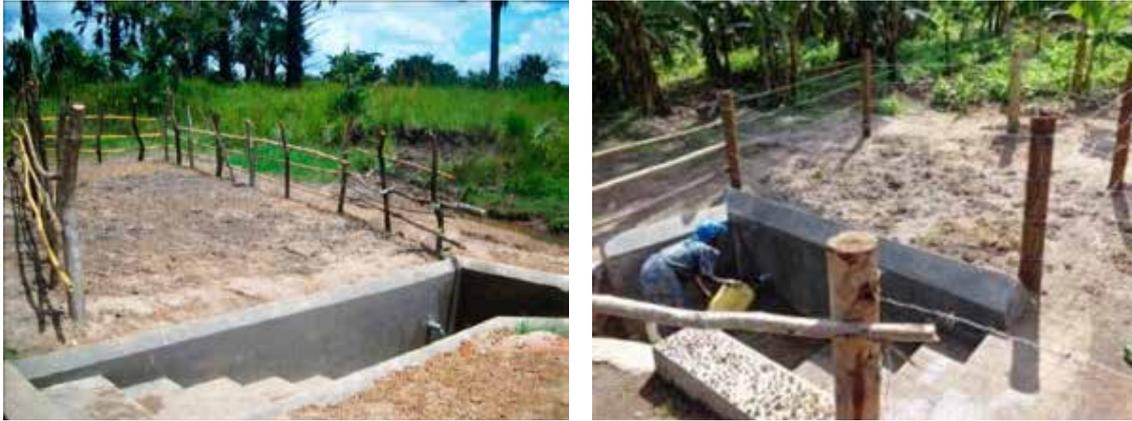
**Figure 9: Medium size protected spring (left) and small size protected spring (right)**
