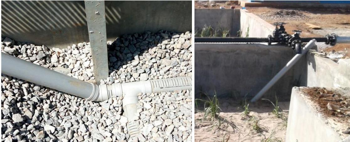
**Fig. 2-13: Drainage system: cleaning and unclogging pipe end**
