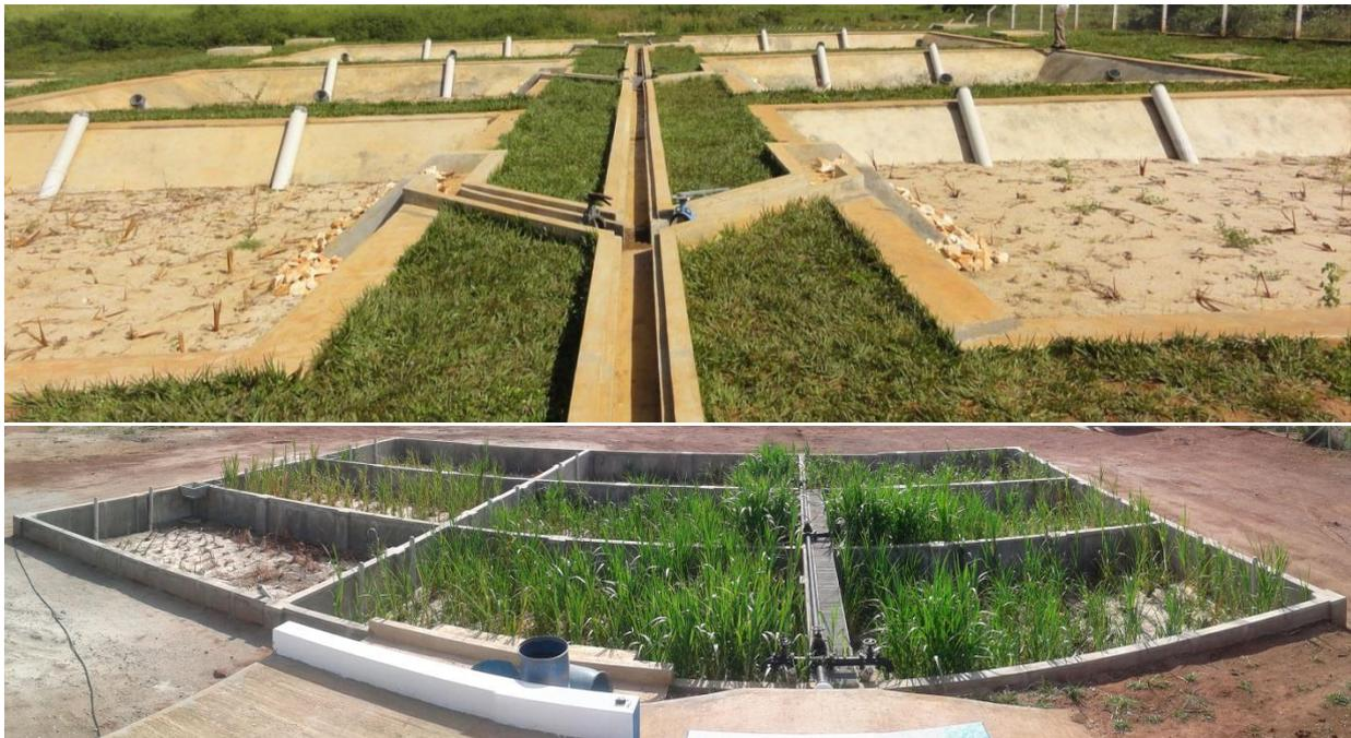
Fig. 2-7: PDB beds construction (on top, separate beds; on bottom, joining beds, i.e. boxes)
