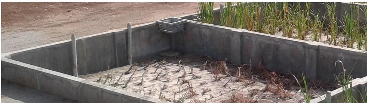
**Fig. 2-6: FS Dumping Area and Pre-Treatment: direct dumping with mobile screen basket**
