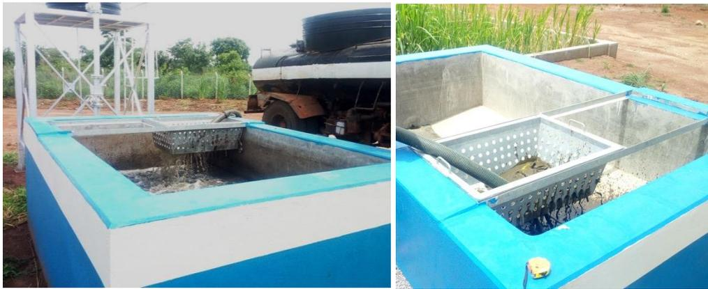
**Fig. 2-5: FS Dumping Area and Pre-Treatment: Apac example**
