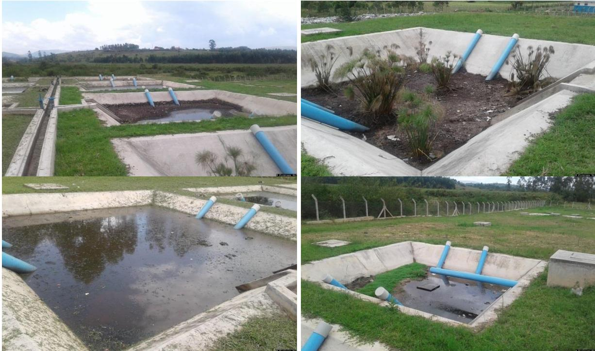
**Fig. 6-5: Ntungamo FSTP: bed overloading and clogging (2018)**
